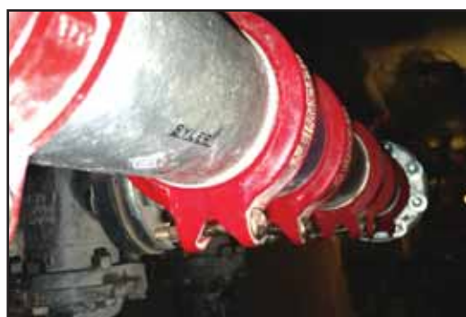
Grooved fitting with plastic lining
